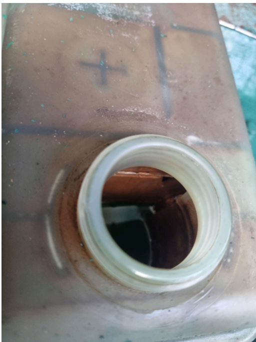
Port engine coolant
